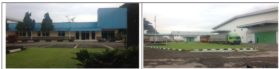
Gambar 4.1 PT. Herlina Indah Indah
