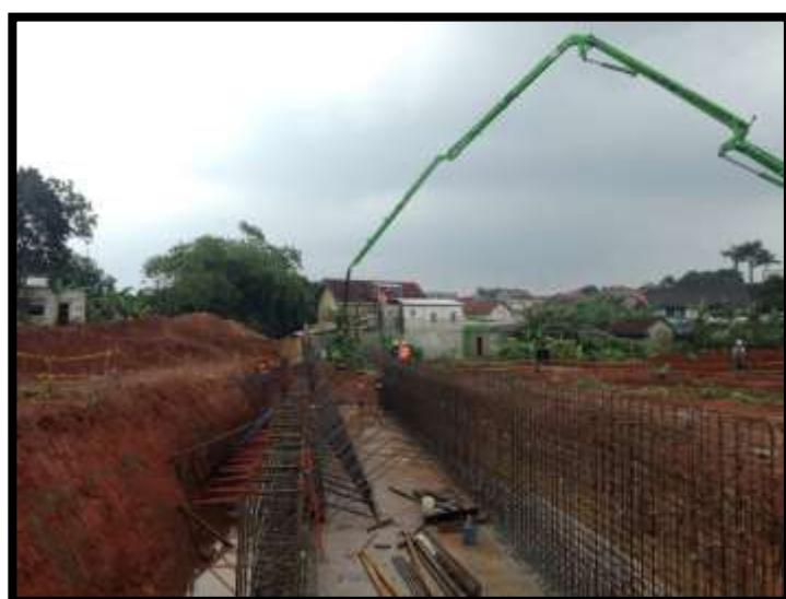
Gambar 2.3 Proses Pengecoran dinding *Box Culvert*
