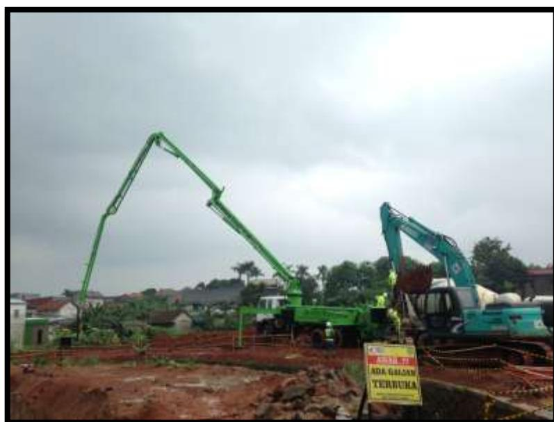
Gambar 2.4 **Concrete Pump**
