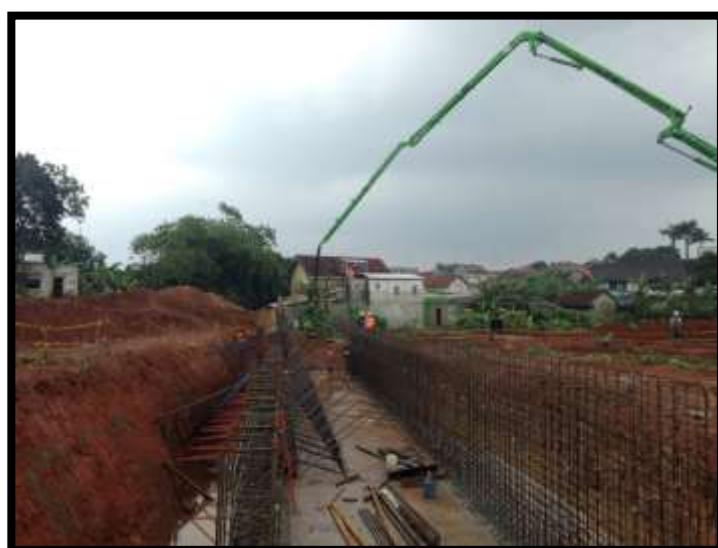
Gambar 2.3 Proses Pengecoran dinding *Box Culvert*
