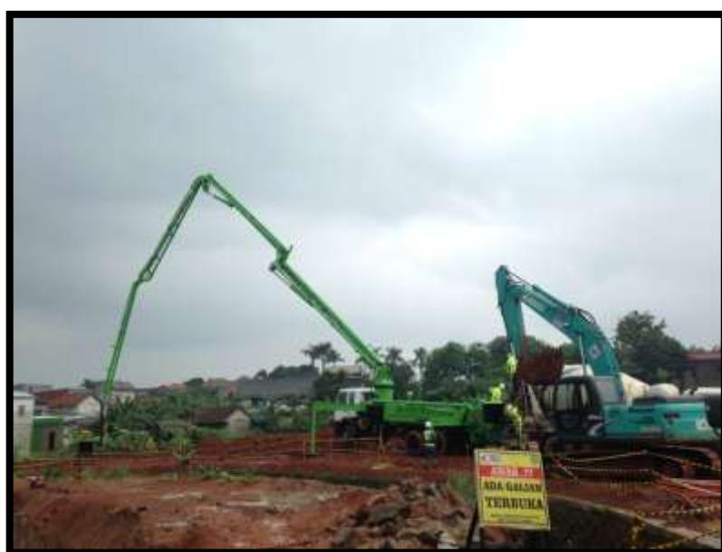
Gambar 2.4 **Concrete Pump**
