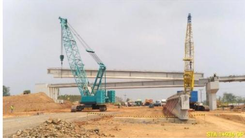
Gambar 2.5 Penegakkan *PCI-Girder*
