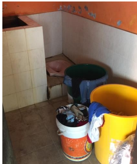
Figure 3 Bathroom condition at school
