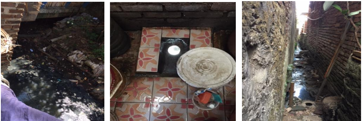
Figure 6 On-site observation (improved toilet with open channel)
